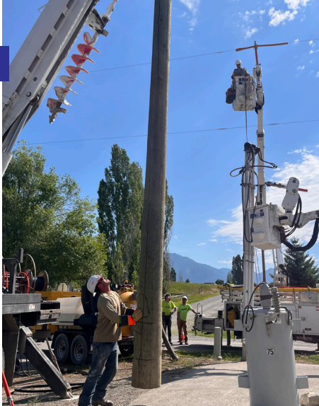
During the power pole replacement.
