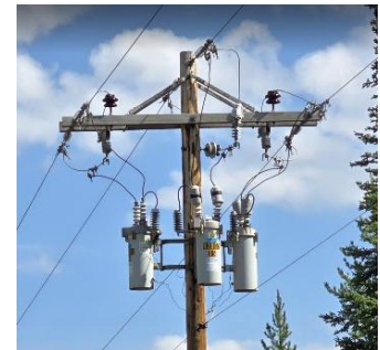
Figure 9 - Hydraulic Reclosers
