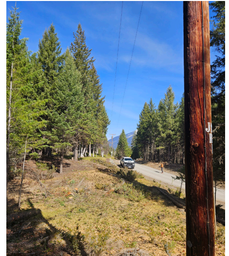
RIGHT-OF-WAY MAINTENANCE WORK
