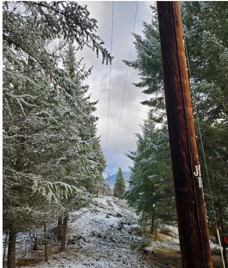
RIGHT-OF-WAY MAINTENANCE WORK
