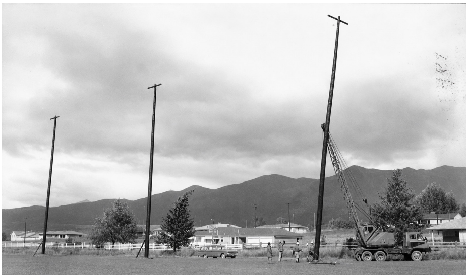
LEC Line Crews install the Eureka Lion's Football Field lights in 1957. | LEC FILE PHOTO
