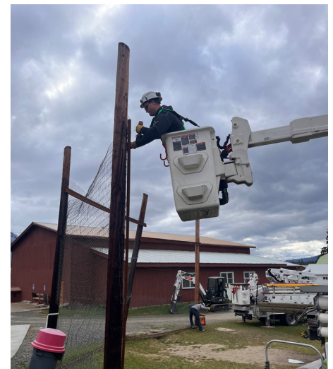
A LEC line crew dismantled and replaced the Fortine School baseball field backstop.
